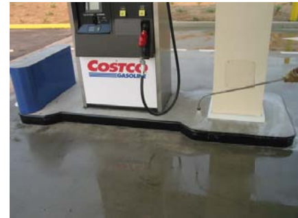
A simple spray application of CMW
